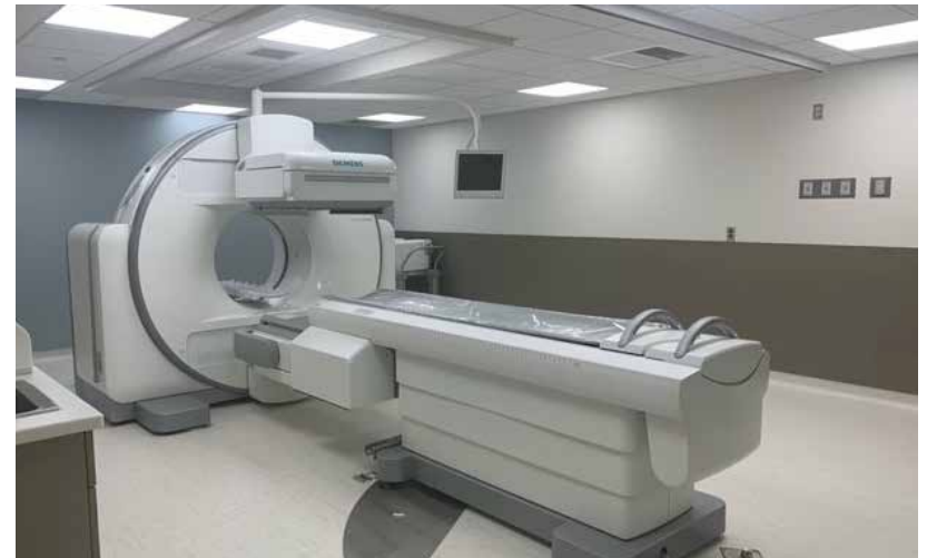
The new nuclear medicine space at Cadillac Hospital features a SPECT CT Nuclear Medicine camera, pictured above.
